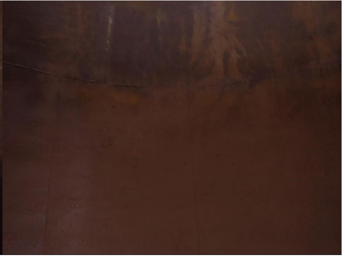
Lower sidewall before washout
