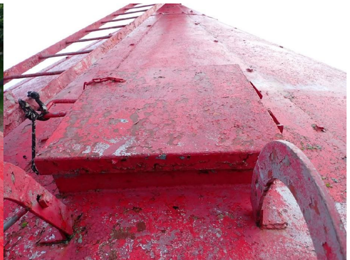
Roof access hatch
