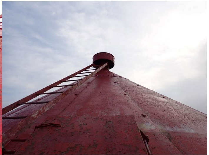
View of tank roof
