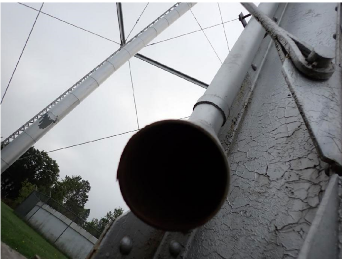
Overflow termination point
