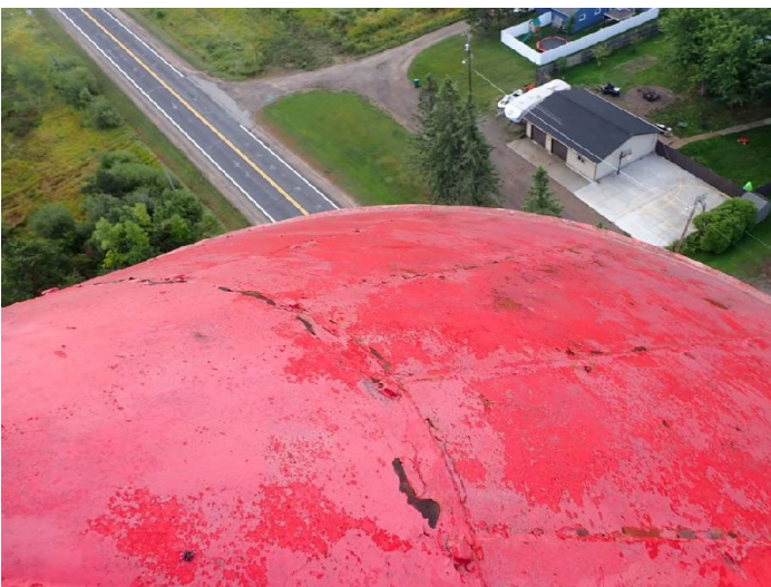
View of tank roof
