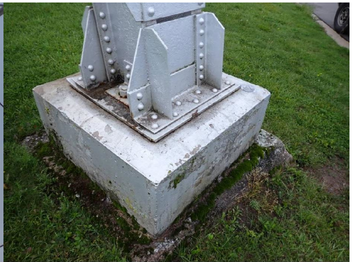
Tank leg and foundation
