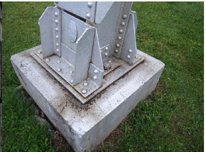
Tank leg and foundation
