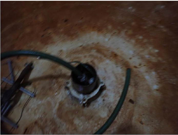
Tank floor after washout
